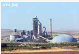
CEMENT PLANT Bucket elevator
